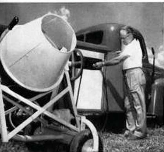
... to power cement mixers ...
